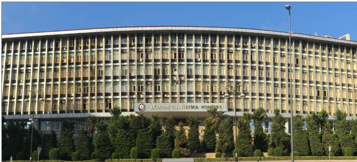
Administrative building of the State Statistical Committee of the Republic of Azerbaijan, Baku
